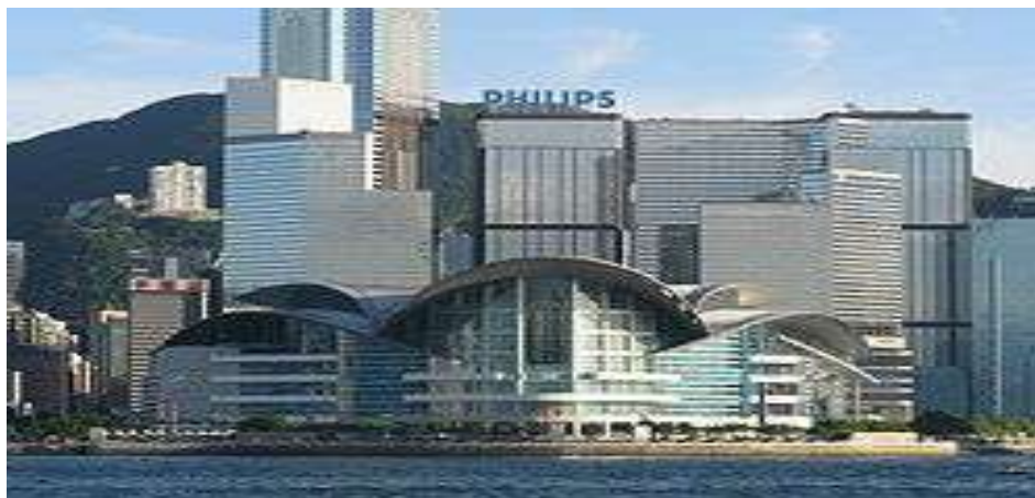
Figure 4.1: Site Photo (Source: http://www.hkcec.com )
